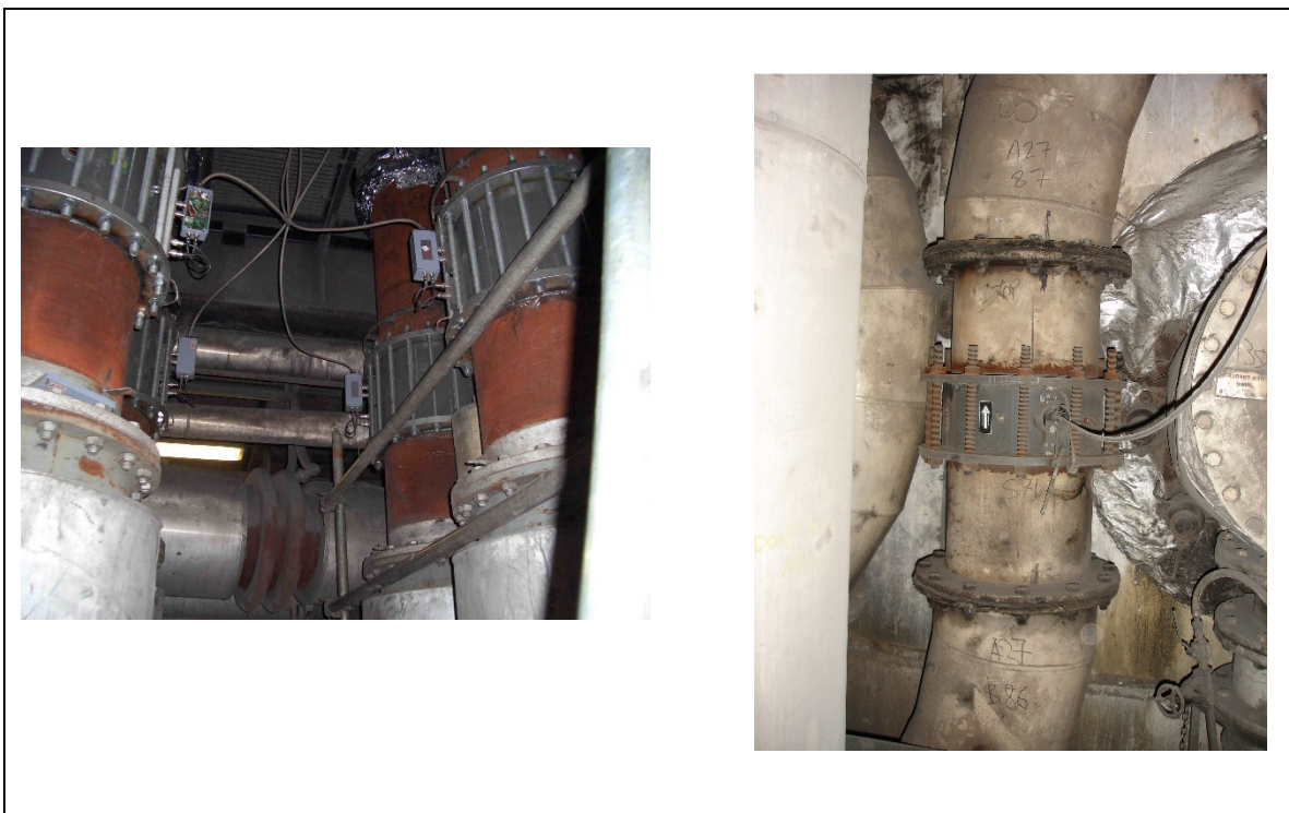
Figure 5 – Examples of vertical installations, left Sensors at same pneumatic distance from upstream bends in vertical, Right , 3 way splits just before burners only allowing very short sections of pipework. Right , remote sensor electronics box used for ease of installation.
