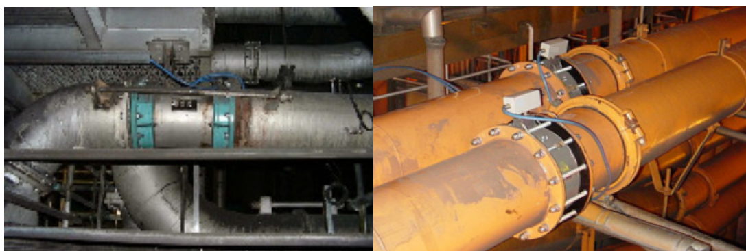
Figure 6 - Sensor for T-fired boiler at beginning of horizontal run to ensure minimal effects from coal deposition. No available horizontal sections of pipe on this boiler configuration.
